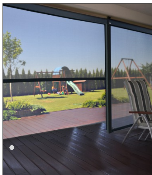
ZIP-78 with fabric EKRAN view from the inside
